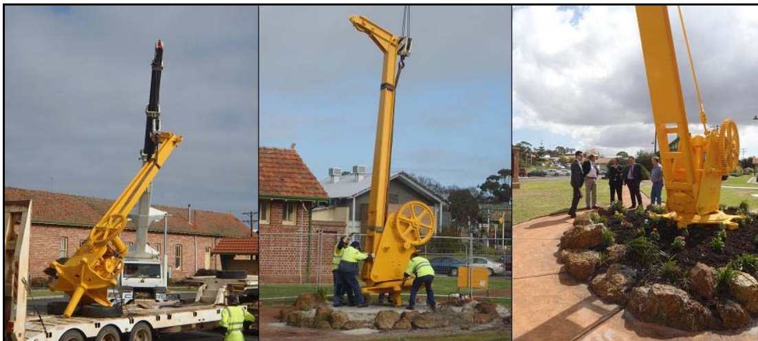
Erection of historic crane
