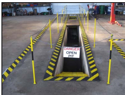
Improved 'Danger' Signage – Depot Inspection Pit
