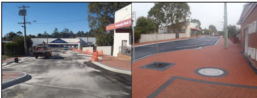
Short Street under construction
