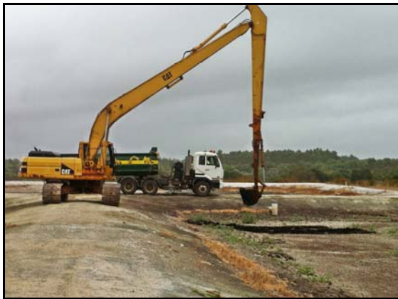
Excavator starting to remove sludge
