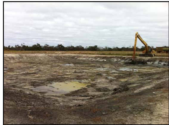
Excavator completing sludge removal
