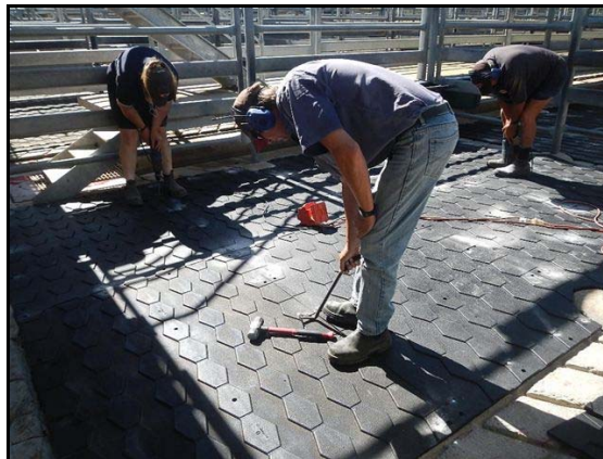
'Surefoot' rubber mats being laid by staff
