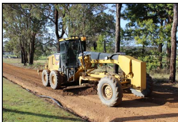
Maintenance Grading - Mount Barker
