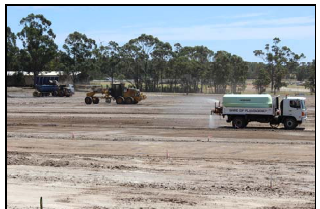
Cricket oval under construction
