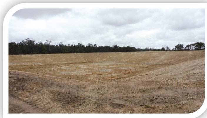
Frost Park Training Track Dam – constructed in February 2017 (Capacity 19 million litres)
