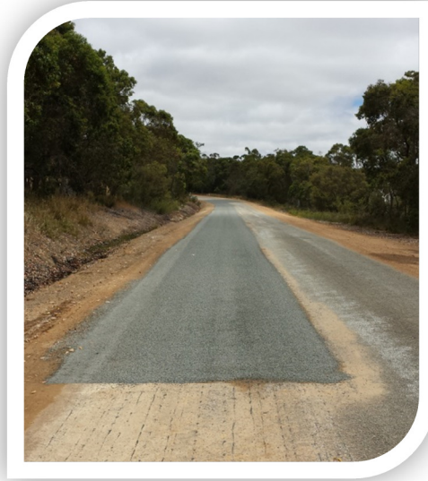
Stabilising repairs to O'Neill Road - December 2016
